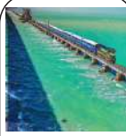
Pamban Railway Bridge
